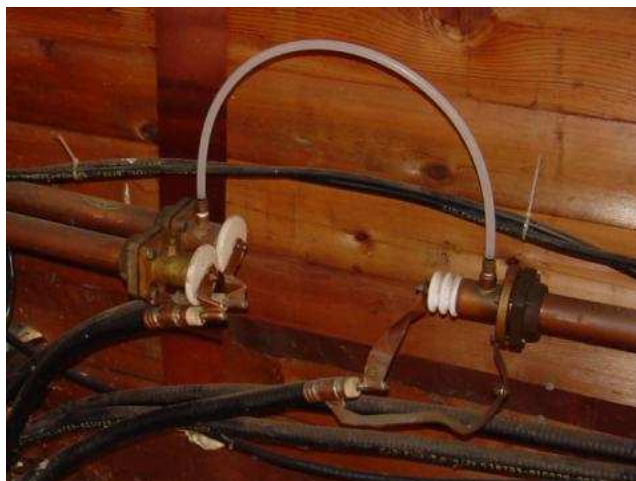
Figure 14.52: Flexible coaxial cables connected to rigid lines.
